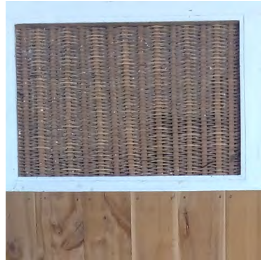
Figure 4. 11 Larger use of wicker-work type on older house type
