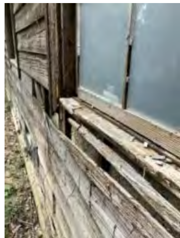
Other instance of damaged clapboard corresponding to hole on the mud wall interior side
