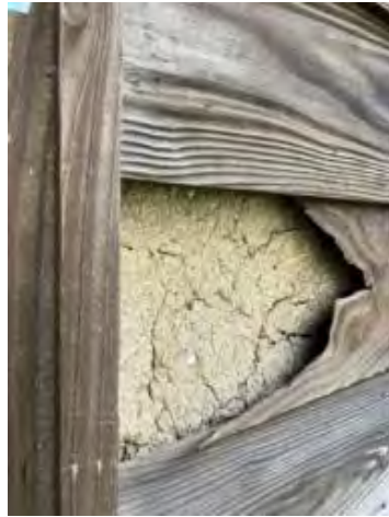
Occurrence of water exposure (outdoor-left) with damage of wall infill
