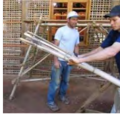
Figure 4. 24 Brazilian worker with takewariki . Split bamboo used for wall grid in the background.(source: Hijioka)
