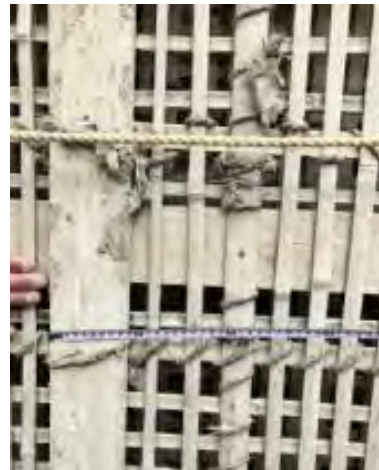
Bamboo grid: take-komai as substrate for mud-wall
