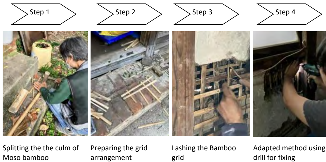
Figure 4. 19 Photographic series: Steps on replacing bamboo grid (take-komai) within adapte technique
