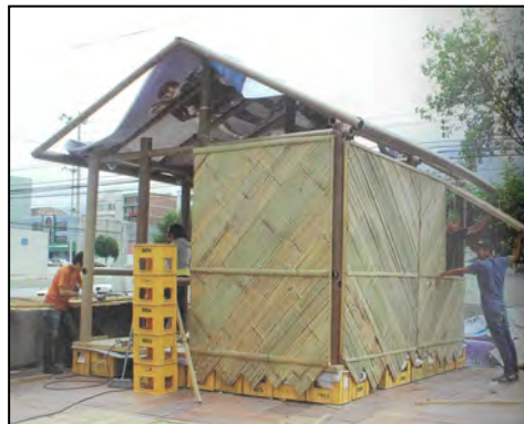
Figure 2. 2 Temporary Bamboo Shelter in Ecuador, designed by Shigeru Ban using flattened bamboo with diagonal arrangement for wall and structural bracing (Ban, 2021)
