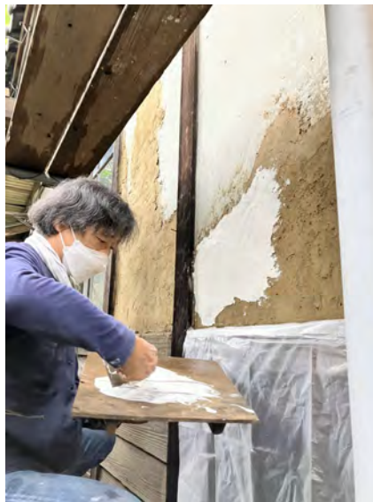
Figure 4. 43 Artist I applying thin layer of white lime ( Shikkui )
