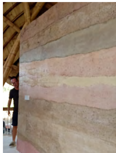
Figure 2. 15 Earth wall plastered with cement plaster to cover damage in Lombok. The damage occurred despite covered by large bamboo roof
