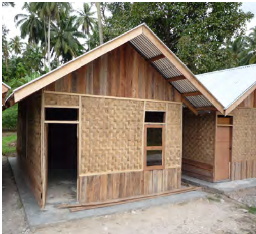
Figure 3. 3 Bamboo wall with timber frame for post-disaster housing in West Sumatra, 2009
