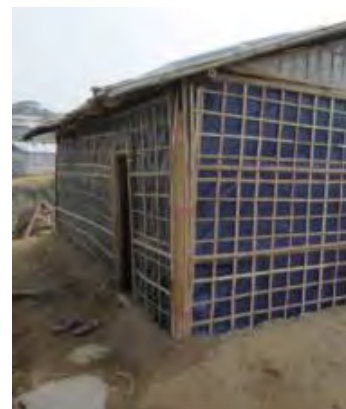
Figure 3. 10 Use of bamboo grid and cladding of bamboo column (source: Kaminski, 2018)
