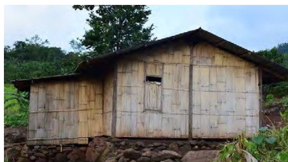
Figure 4. 33 Flattened bamboo wall within dry method, suggested more prevalent in Sikka, Flores, Indonesia after the 1992 earthquake (source: cendananews.com)
