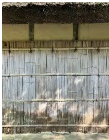
Figure 4. 33 Use of flattened bamboo for cladding (Shitami-itabari) in traditional Japanese house
