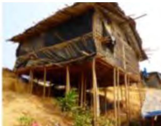
Figure 3. 9 Use of bamboo for pier, wall and roof (source: Kaminski, 2018)
