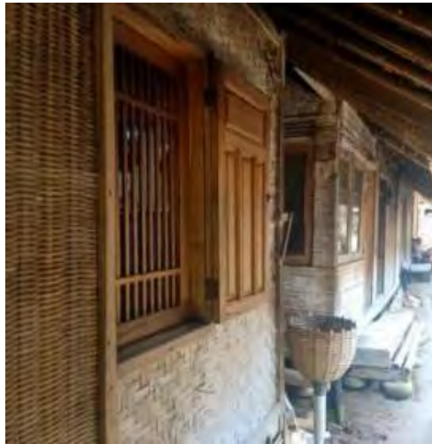
Figure 4. 10 Use of woven wicker-work (kitchen-left) and plait-work type
