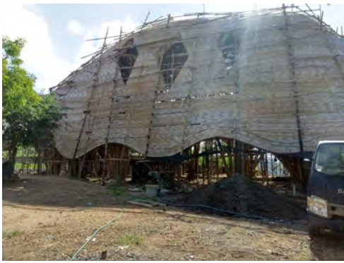
Figure 2. 5 Large bamboo roof structure built by workers from Belega village, Bali.
