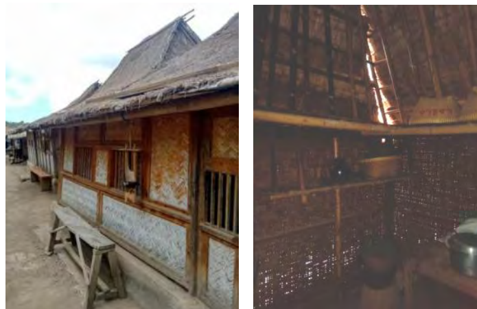
Figure 4. 7 Exterior and Interior view of the woven-plait work bamboo wall
