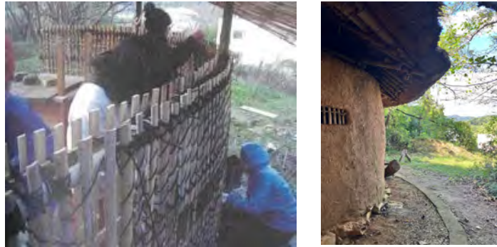
Figure 4. 21 New construction method of Mud-wall with adapted technique for ‘Tsuchi-no-Ie’ (Source: Inoue, 2021)
