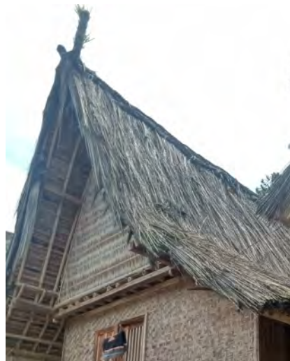
Figure 4. 38 Wicker work wall protected by roof eaves in Naga village older building
