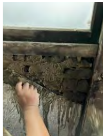
Hole below window partially filled with ara-nuri (rough wall mud)
