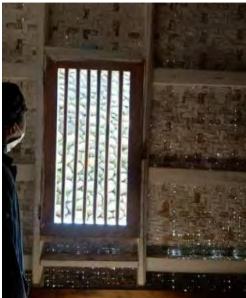
Figure 4. 12 Interior view of the house with plait-work type, also visible are the lime plaster and pores between the tight weave
